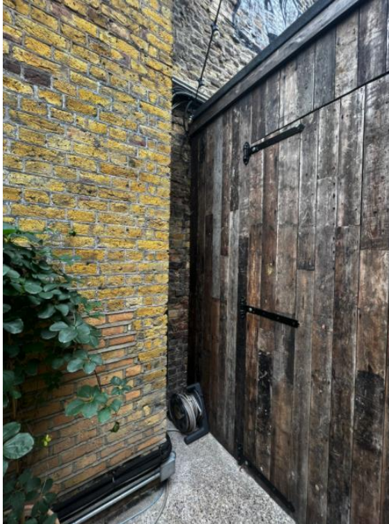
Fig 1 Return behind the wall.
